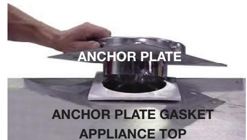
**ANCHOR PLATE FOR A FACTORY BUILT CHIMNEY**
